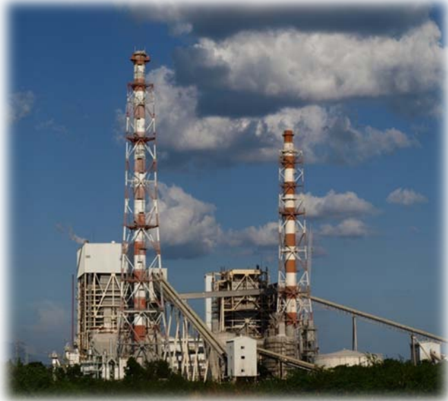
600MW Coal-Fired Power Plant Calaca, Batangas
